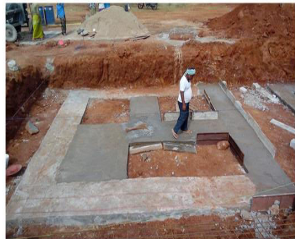
P.C.C foundation of building
