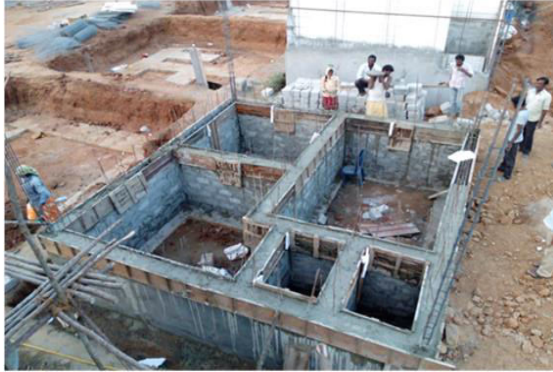
Basement up to plinth level
