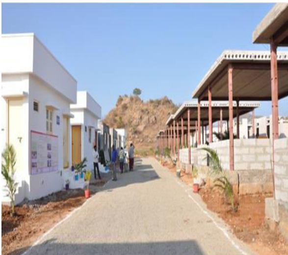
Final view of building site
