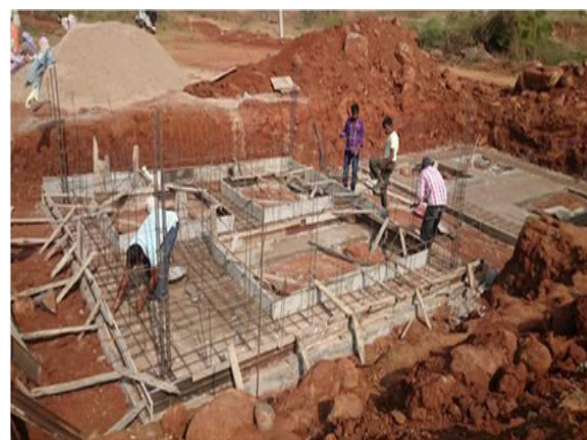
placing reinforcement for raft foundation
