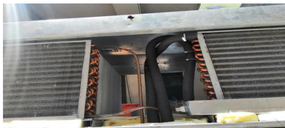
Figure: Copper pipe welding.
