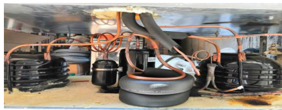
Figure: Refrigerant filling.
