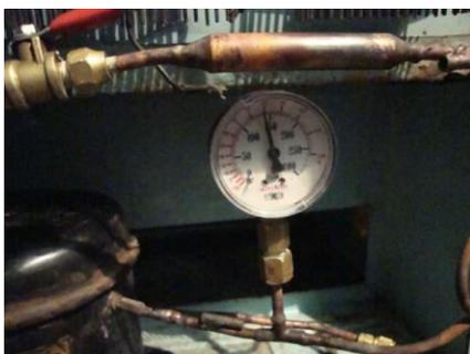
**Fig 4.3 Discharge pressure gauge**
