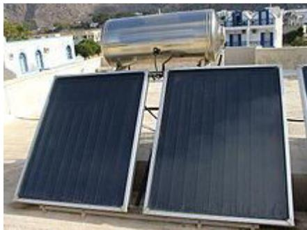
Figure 1: Flat plate thermal device for water heating deployed on a flat roof.
